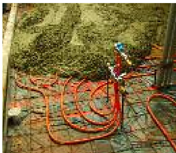
RadiantPEX-AL stays where you want it, making tie-down easier.
